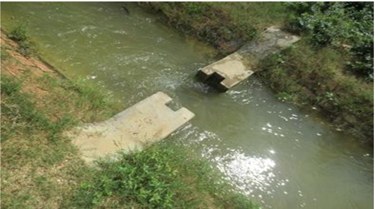
Figure 17: Sample check structure proposed for canal
