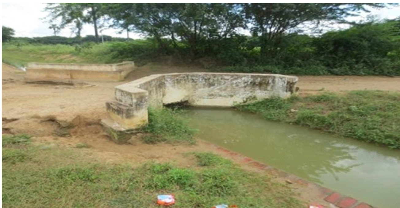
Figure 18: A sample of proposed culvert for crossing drain and road
