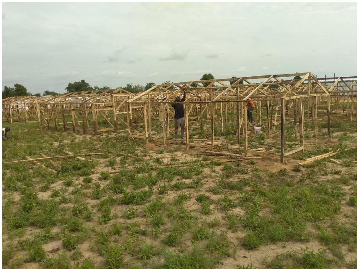
Photo: Mercy Corps USAID funded Emergency shelter construction in Damboa LGA. 2019
