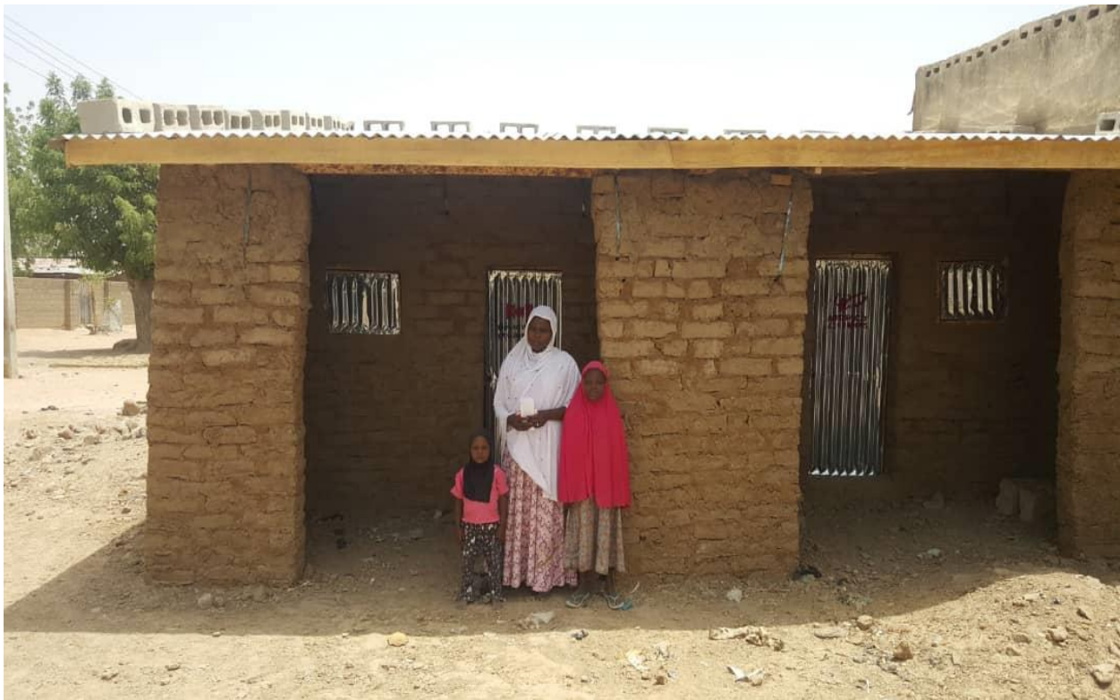
Photo: A two-room mud bricks shelter constructed by Mercy Corps in Dikwa in March 2019
